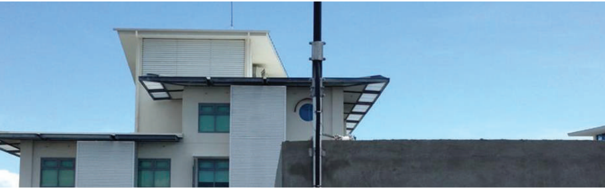
LPI air terminal protecting a hospital in India
